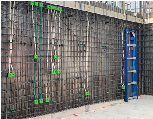
Images 2 & 3: Spelsberg IBT enclosures are suitable for installation in in-place concrete and prefabricated elements.
