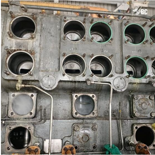
Image 1: The compressor was disassembled in the local service center for a technical assessment.
