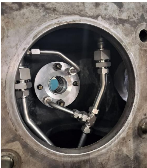
Image 2: The new rod packing solution significantly improved the compressor's reliability.
