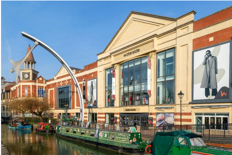
Image 1: The finished project delivered an enduring, high-quality facade.
