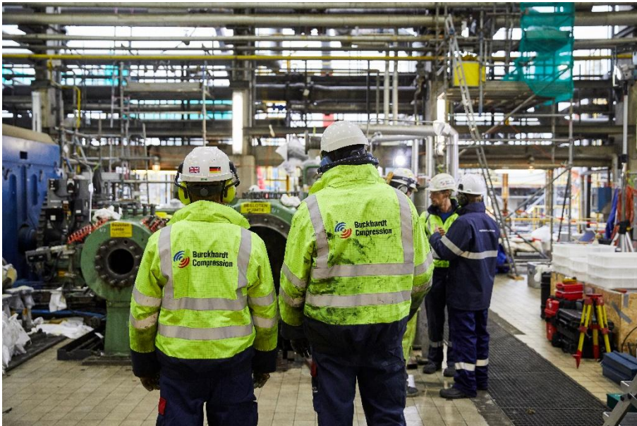
Image 2: Smooth on-site overhauls are the culmination of in-depth planning and effective organization.
