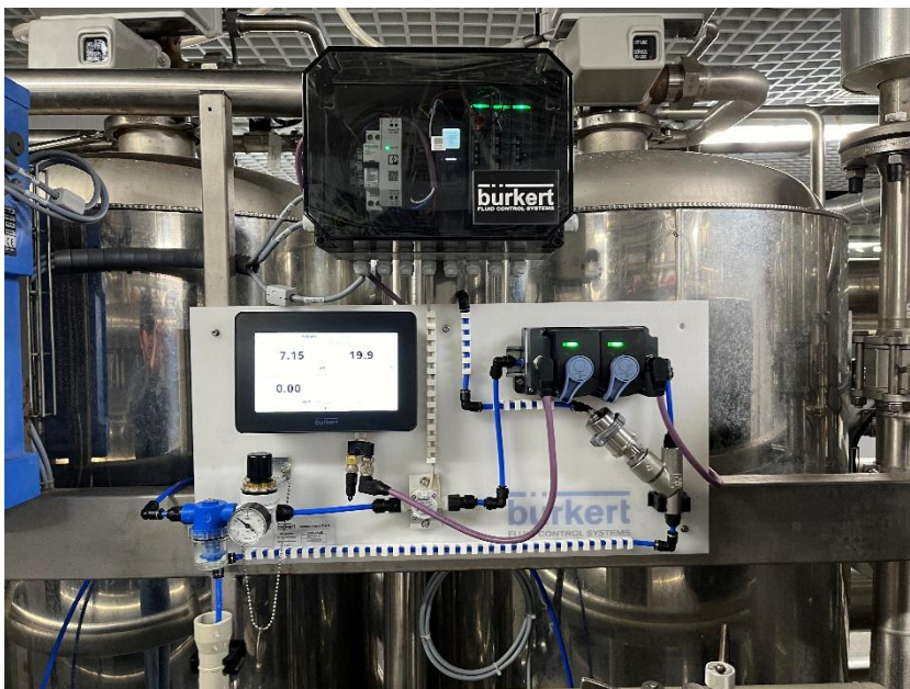
Image 2: An example of Bürkert's compact solutions for measuring free-chlorine after a granular activated carbon filter.
