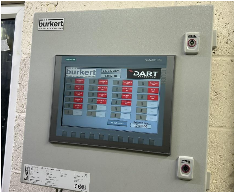
Image 1: The centralised control panel includes an HMI touch-screen to enable individual machine management.
