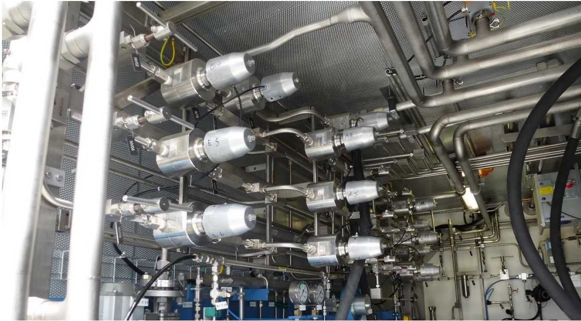
Image 1: Bürkert offers a range of valves specifically designed for high-pressure and ultra-high-pressure hydrogen applications.
