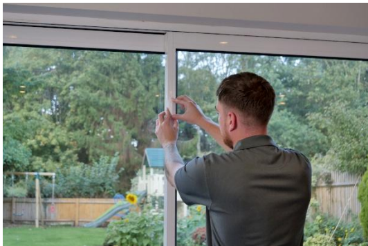
Image 5: Installation causes minimal mess as most of the sensors are completely wireless and the components are Wi-Fi enabled.
