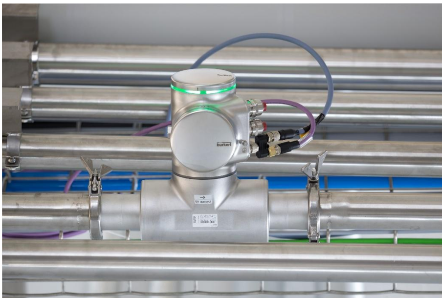
Image 2: The FLOWave is a multi-parameter sensor that saved space and delivered at least a 40% cost saving compared to the Coriolis alternative.
