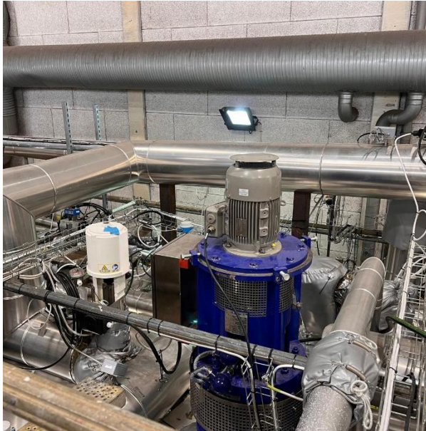
Image 1: The installation phase of Sulzer's advanced pumps for Hyme Energy's pioneer molten hydroxide salt energy storage system.
