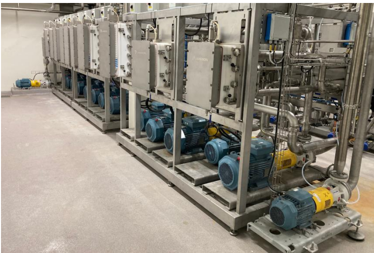
Image 4: SNS pump units on starch washing
