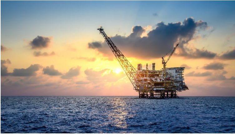
Image 1: Local engineering support is important for offshore platform construction and operation
