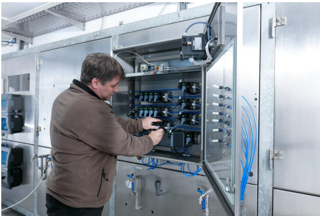
Image 2: The Type 8906 Online Analysis System enables modular integration of sensors such as pH, free-chlorine, and turbidity, which can be monitored remotely via GSM modules.
