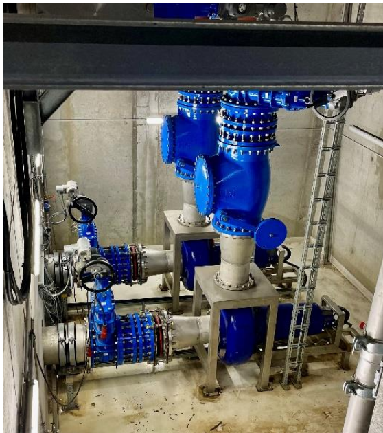
Image 2: The XFP pumps were mounted horizontally on sliding carriages in order to simplify maintenance.
