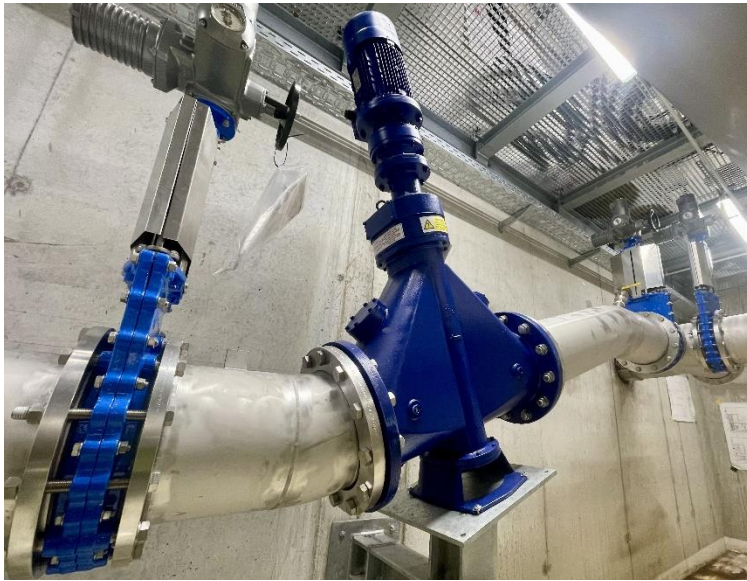
Image 3: The Muffin monster inline grinder ensures continuous pump reliability and extended service life.
