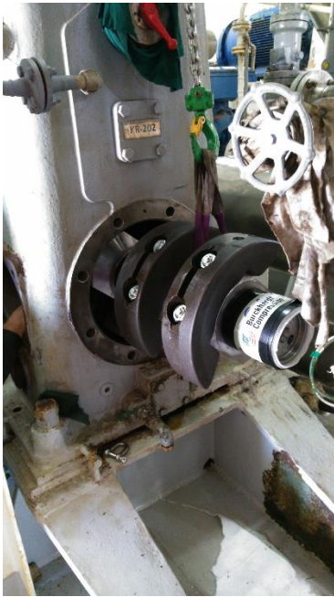
Image 3: The new, reworked crankshaft being installed.
