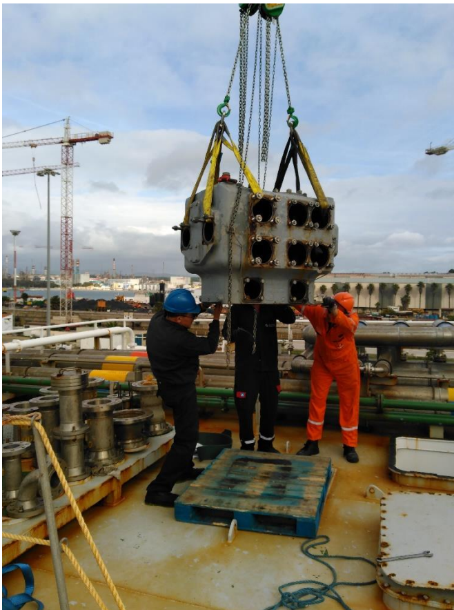
Image 2: The damaged cylinder was machined to accept over-sized components.
