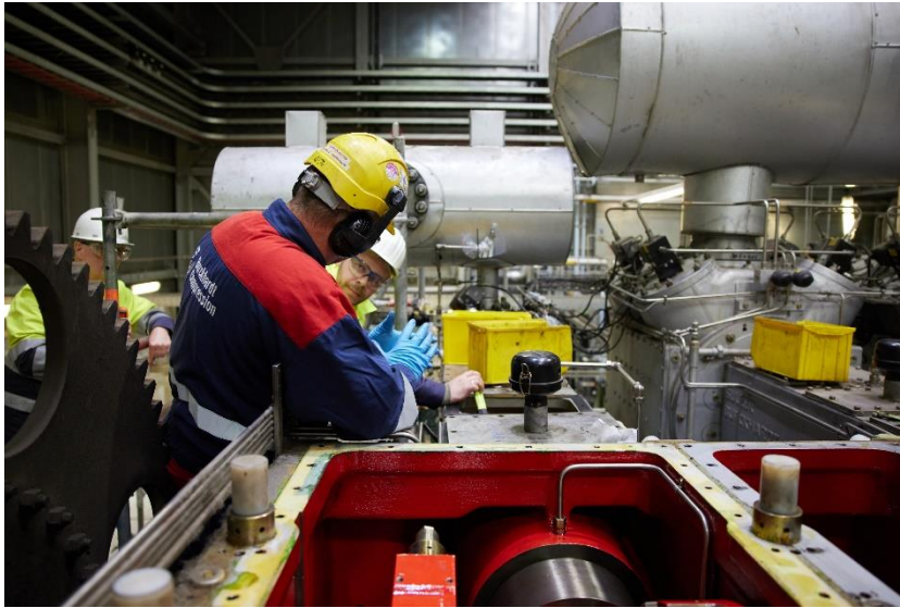
Image 1: Careful inspection of compressor components, including sealing systems, is essential to identifying leaks.
