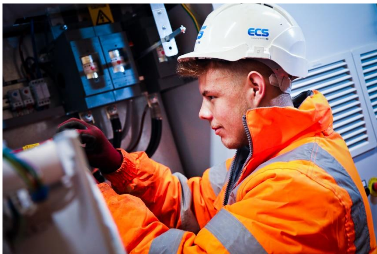
Image 2: ECS are specialists in the distribution, installation, and maintenance for a range of Archimedes screw pumps and provide essential support to Severn Trent Water's screw pump assets
