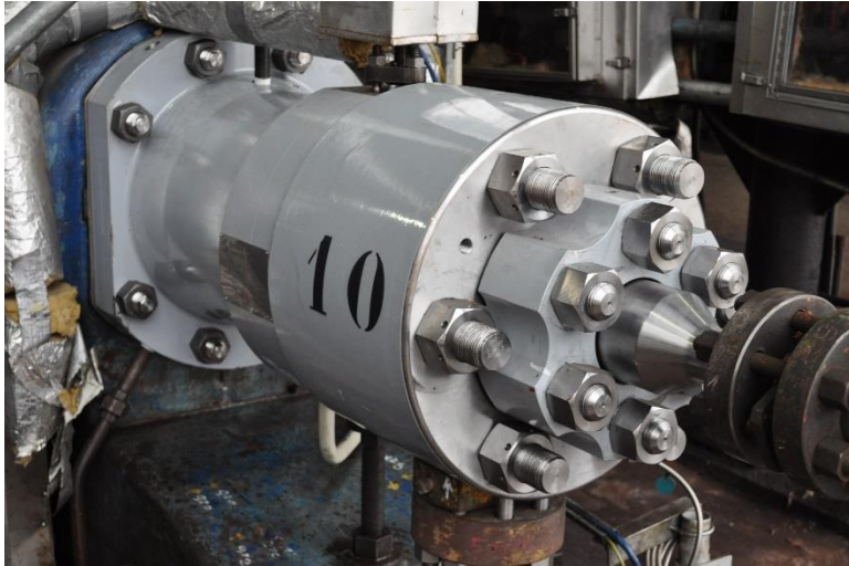
Image 1: The new cylinder after installation.
