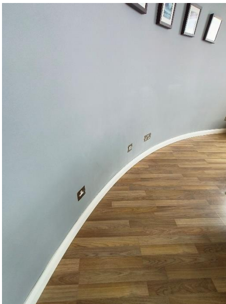
Image 4: Shadow gap beads are suitable for curved walls
