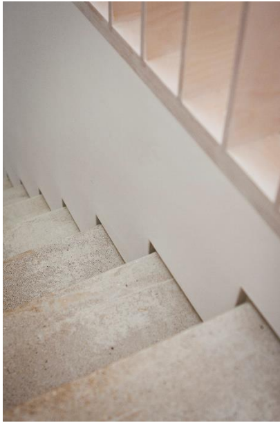
Image 3: Shadow gap beads in place on a staircase
