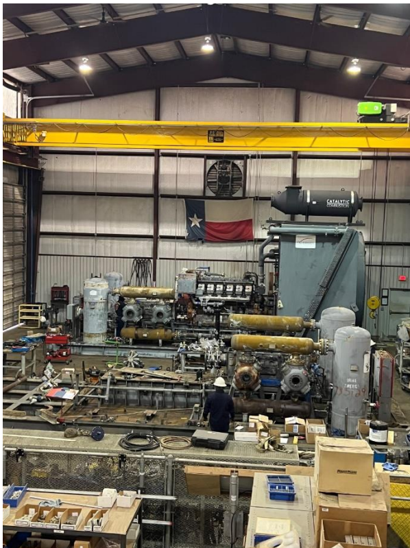
Image 2: Compressor repairs at Kilgore service center
