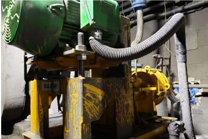
Image 3: EMW slurry pump at the site
