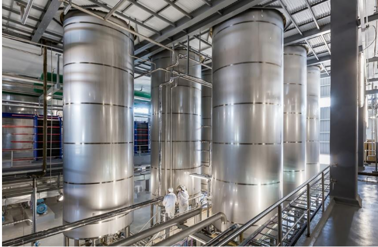
Image 1: Yeast fermenters at Refineria del Centro site
