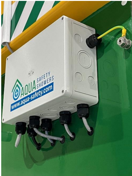
Image 1: Aqua Safety Showers partnered with Spelsberg UK junction boxes that protect terminal connections.
