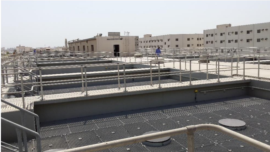
Image 1: The original 20 sand filter basins were converted to DynaSand filters
