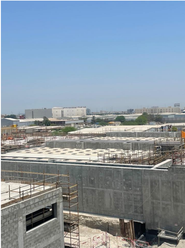
Image 3: The latest expansion project used purpose-built concrete basins
