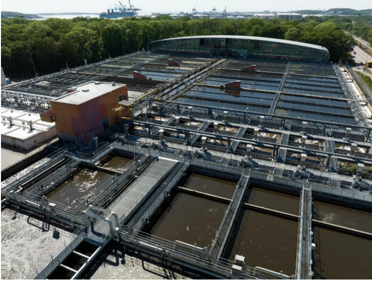
Image 1: The wastewater treatment plant has an average inflow of 4'000 liters per second
