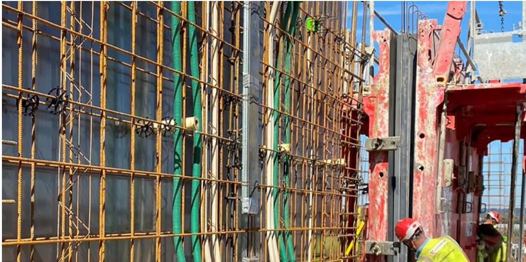
Image 1: Legendre UK uses the IBT range from Spelsberg to build modular homes.
