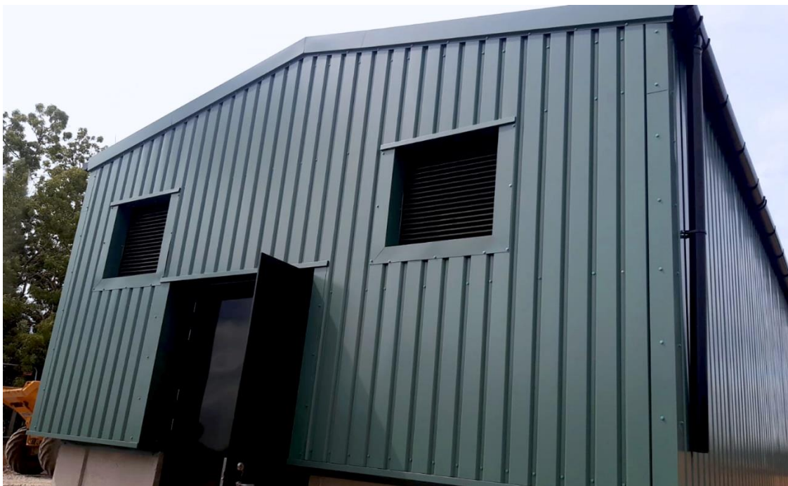
Images 1 & 2: New pump station built at Mundford Road Reservoir by ECS
