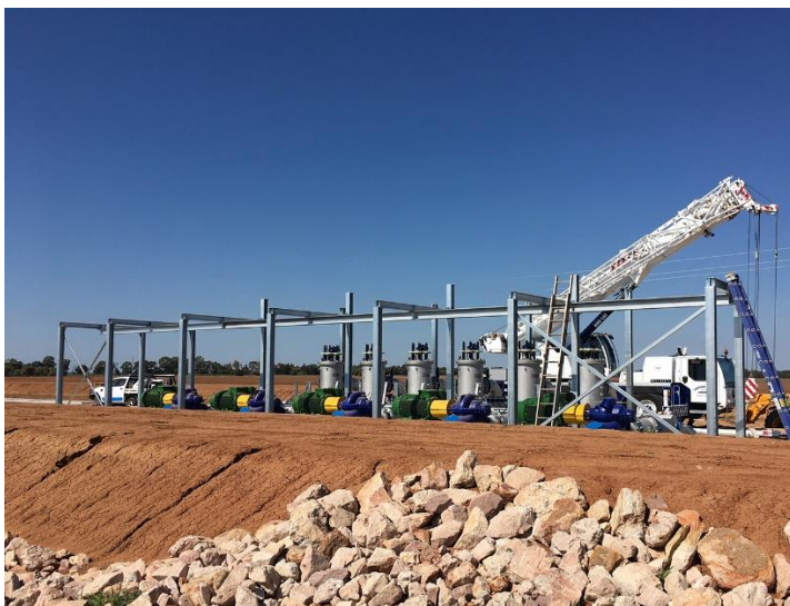
Image 2: Sulzer delivered 16 pumps installed across the three pumping stations
