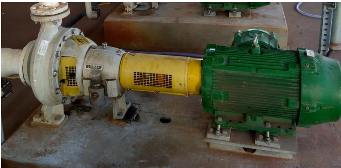
Image 2: SNS3-80 pumping unit for anhydrous ethanol
