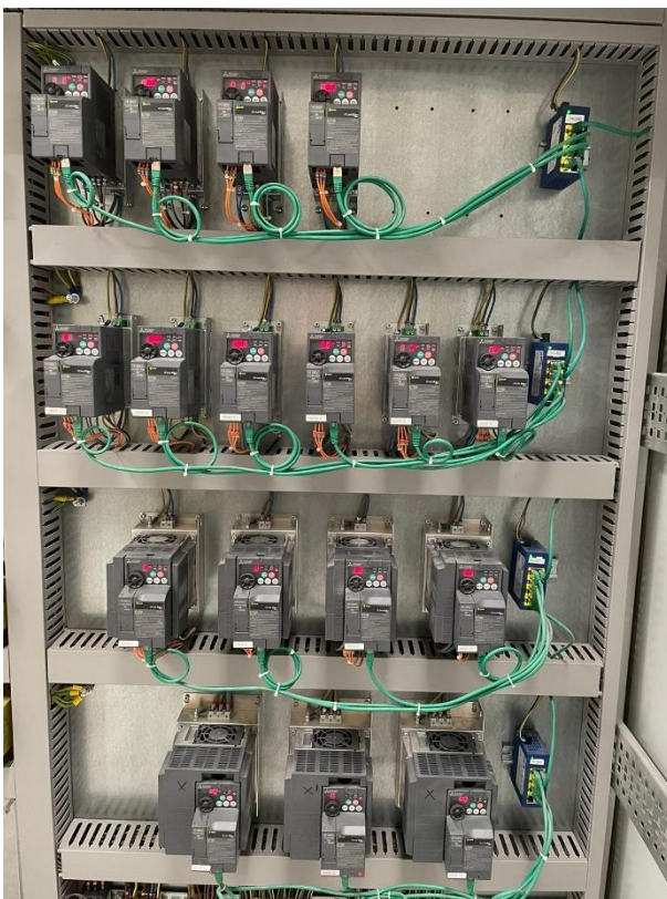
Image 4: The new door press application line was is run by 19 Mitsubishi Electric's FR-E series VSDs. [Source: Mitsubishi Electric Ireland]
