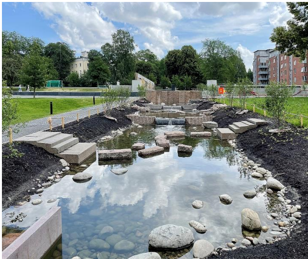
Image 1: Sulzer's pump package operates around the clock from Spring until Autumn
