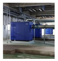
**Image 2:** Six HST 20 turbocompressors from Sulzer were chosen to replace eight units at Derby Sewage Treatment Works to reduce the risk of downtime.
