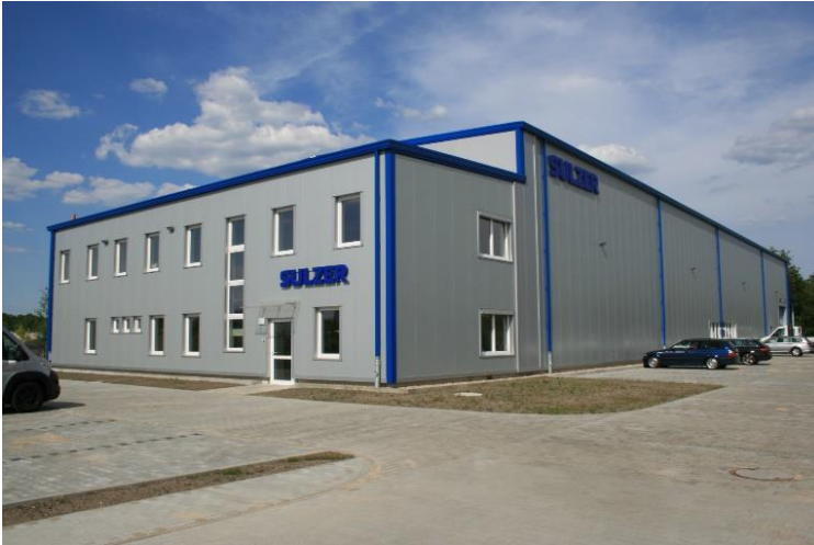
Image 1: Sulzer has announced the opening of its purpose-built Lausitz Service Center
