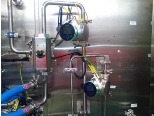
Image 1: The FLOWave offers a very compact footprint, a key priority in this project
