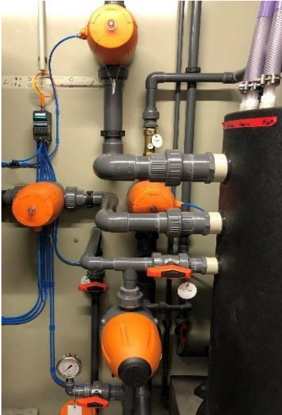
Image 1: The 8653 used in these pilot plants are IO-Link enabled and do not require Communicator to transfer settings.
