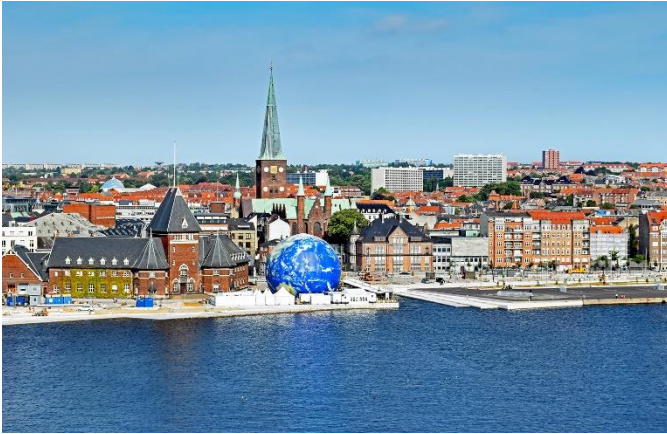
Image 1: Sulzer has completed the first in a series of wastewater pumping stations for a Danish municipality. (shutterstock_686737981)
