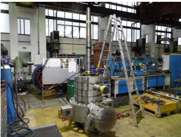
Image 4: From the initial stoppage of the pump to recommissioning, the whole project was completed in nine and a half weeks
