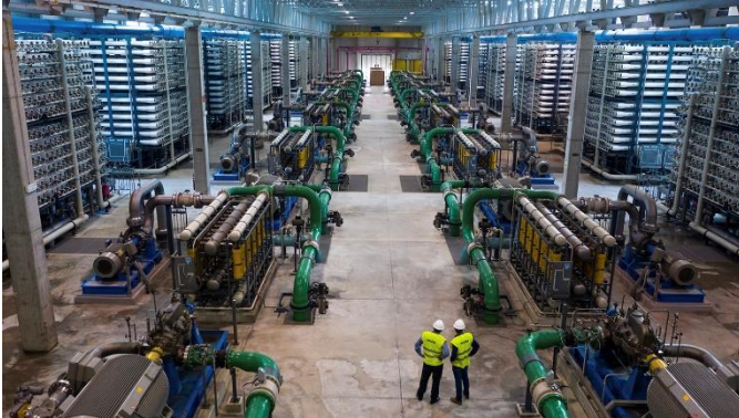
Image 1: Pump efficiency increases with larger RO trains
