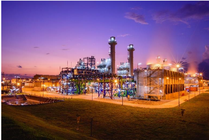
Image 1: Sulzer has a long-standing relationship with the French power plant, being involved with the pumps at the facility for many years
