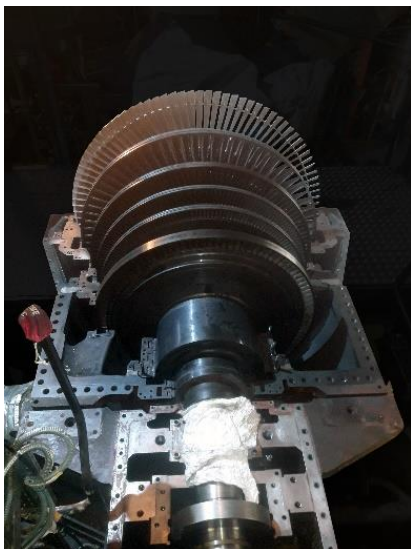
Image 2: Sulzer was awarded the contract to refurbish the steam turbine, the gearbox and the pump it was driving, to be completed within the six-week window
