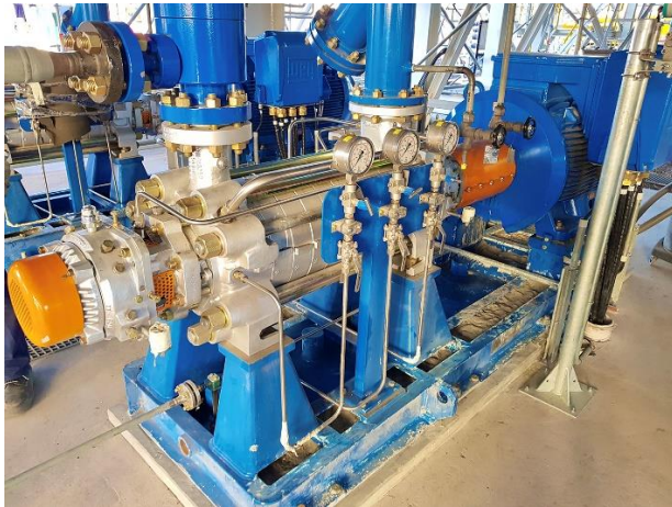
Image 1: Sulzer's boiler feed pumps have become a popular choice for Argentinian power plants
