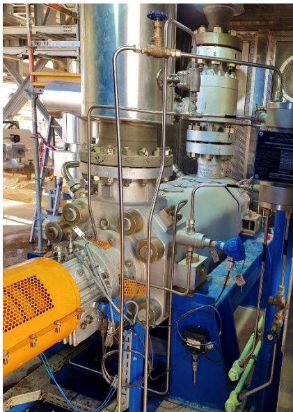
Image 2: Every pump was delivered with all the required instrumentation and commissioned with assistance from Sulzer personnel
