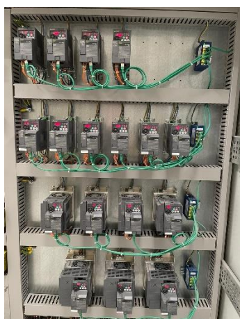
Image 4: The new door press application line was is run by 19 Mitsubishi Electric's FR-E series VSDs.
