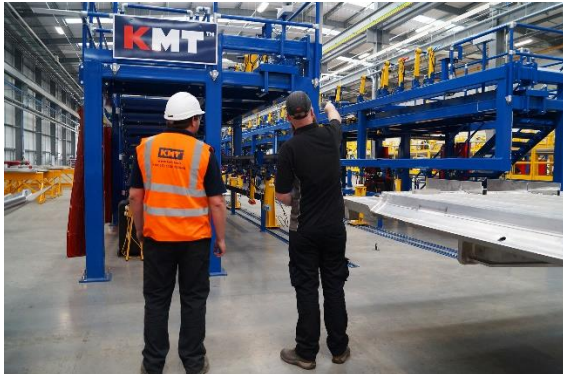
Image 1: KM Tools 'Smart Jig' installed onsite at Hitachi Rail in Newton Aycliffe
