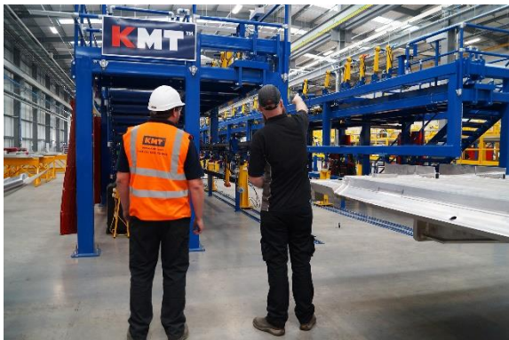
Image 4: KMT experts can provide installation and maintenance services to ensure maximum uptime for production equipment
