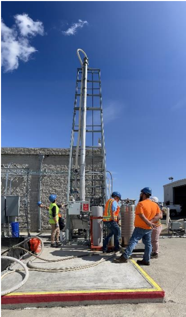
Image 3: CO 2 absorber column using structured packings, distributor and demister.
