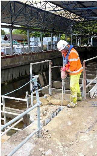
Image 3: The civil infrastructure at the site has also been comprehensively overhauled
