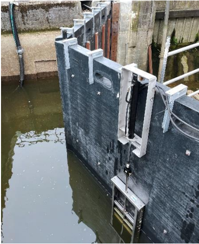
Image 6: FRP lock gates are essentially maintenance free, with the lifespan of an FRP panel at least 100 years
