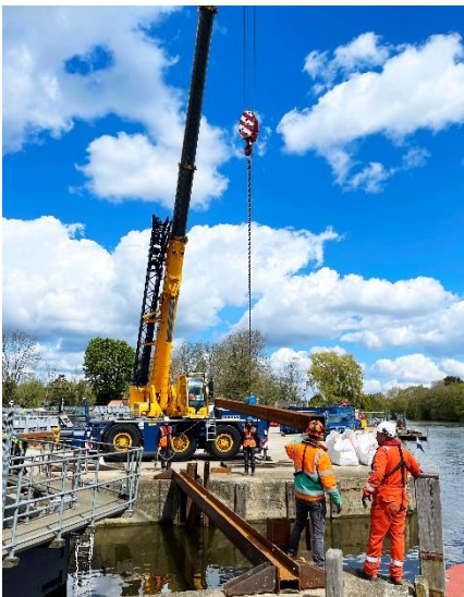
Image 2: The new gates were fitted on behalf of the Environment Agency
