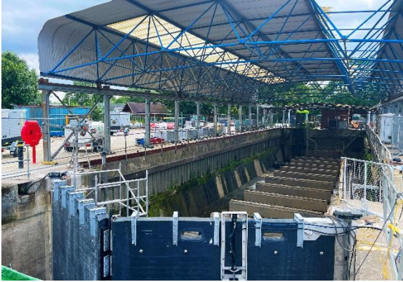
Image 1: ECS has installed the UK's first ever set of FRP lock gates on the River Thames at Sunbury Dry Dock
