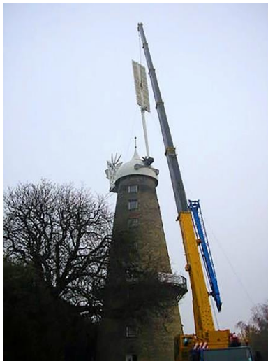
Image 3: The fitment of the blades to the 100 ft high mill completed the restoration project.
