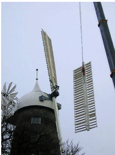
Image 2: The blades were fabricated from profiled plates, which were welded together to form a continuous section.
