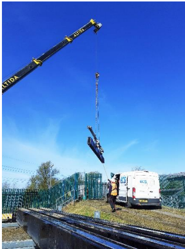
Image 2: The ballast tanks were fitted on behalf of the Environment Agency
