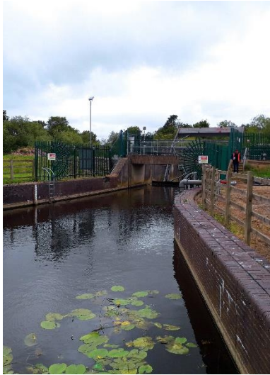
Image 1: ECS has completed the overhaul of the radial gate at Pillings on the River Soar in Leicestershire
