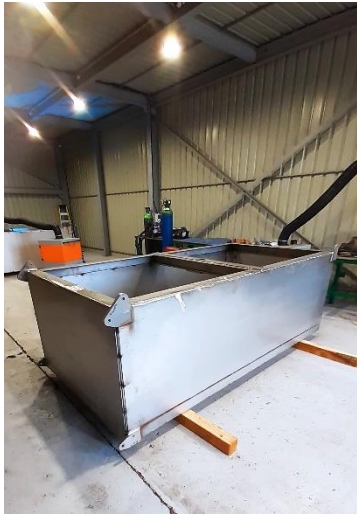
Image 4: The new stainless-steel ballast tanks will greatly reduce future maintenance requirements at the site
