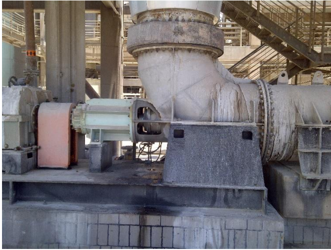
Image 1: Axial flow pump type CAHR1000F running at the site.
