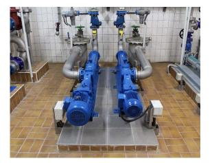
**Image 1:** Bauer Gear Motor has collaborated with Allweiler, combining highly efficient permanent magnet synchronous motors (PMSMs) with Allweiler progressive cavity pumps, at Stendal wastewater treatment plant in Germany.
