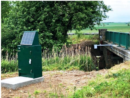
Image 1: ECS upgrades River Glen level sensor with solar powered system
